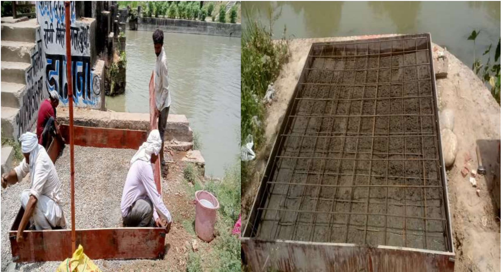
PORTA CABIN FOUNDATION WORK
