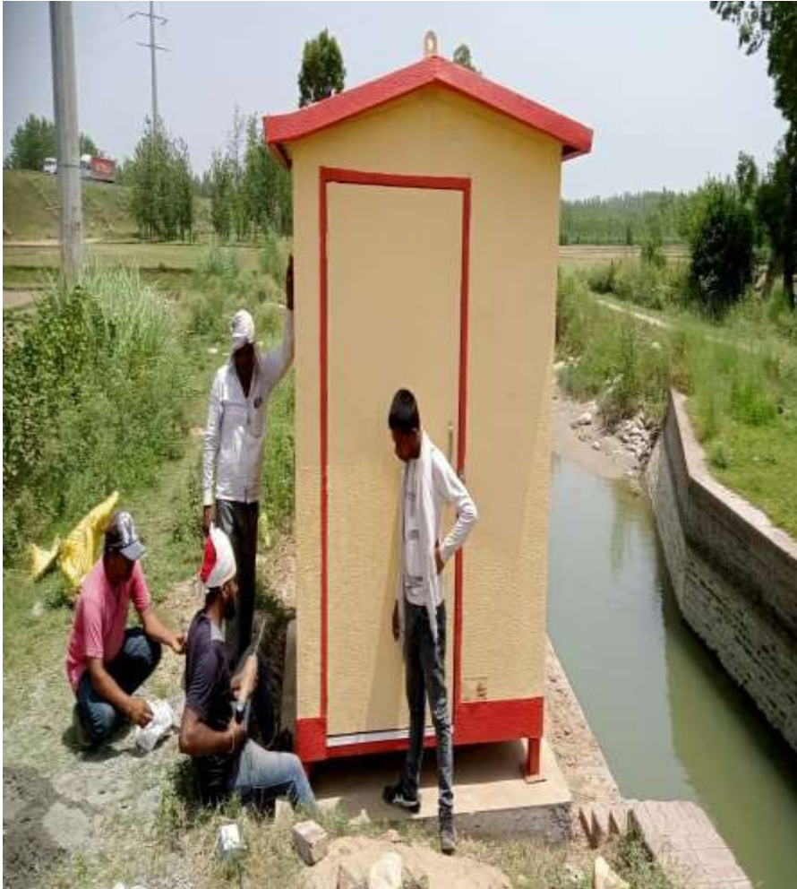
PORTA CABING INSTALLATION WORK
