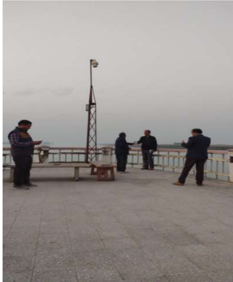
PTZ CAMERA INSTALLATION WORK AT BARRAGE UPSTREAM
