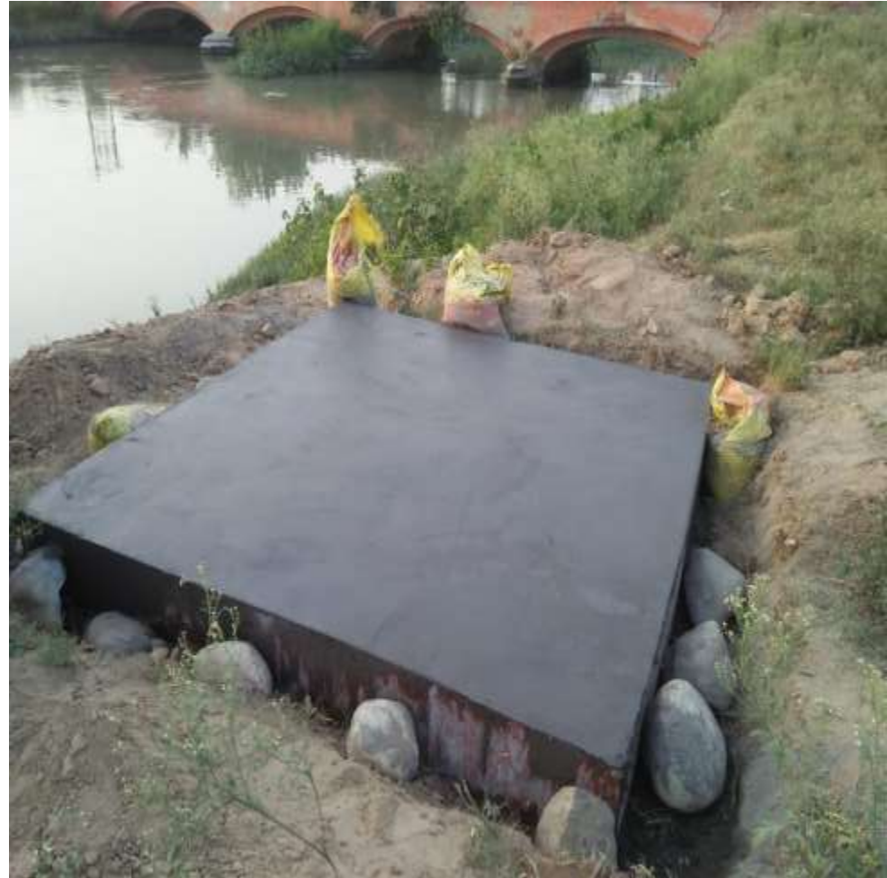
PORTA CABIN FOUNDATION WORK
