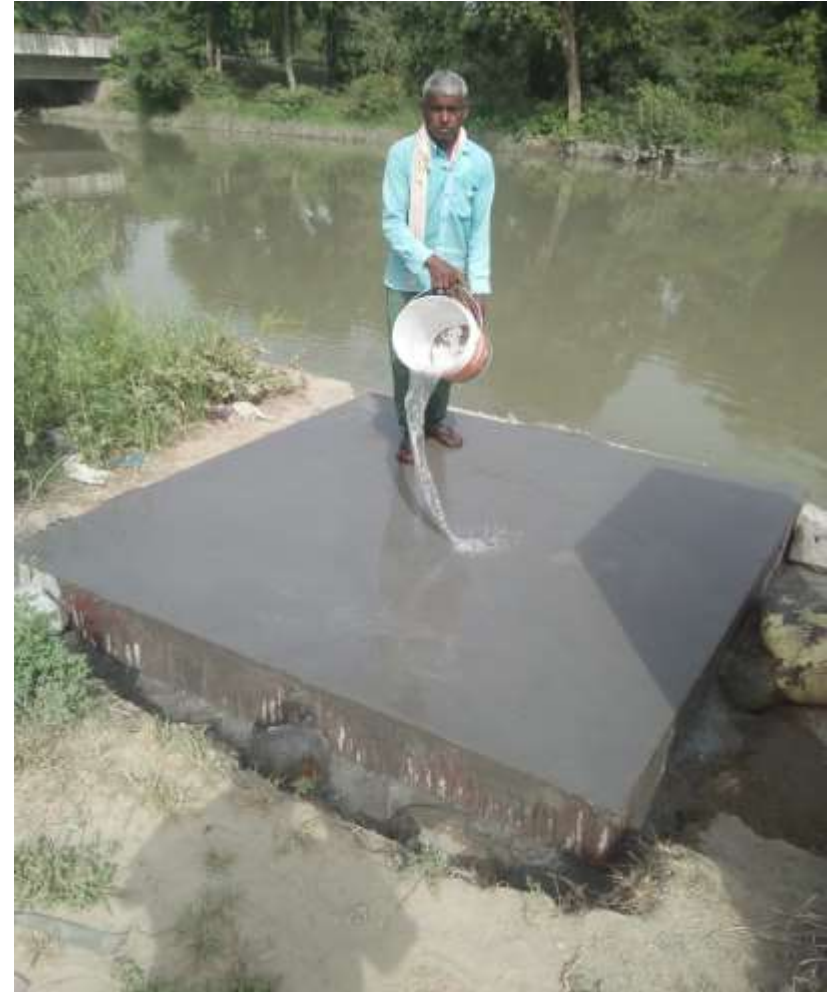
PORTA CABIN FOUNDATION WORK
