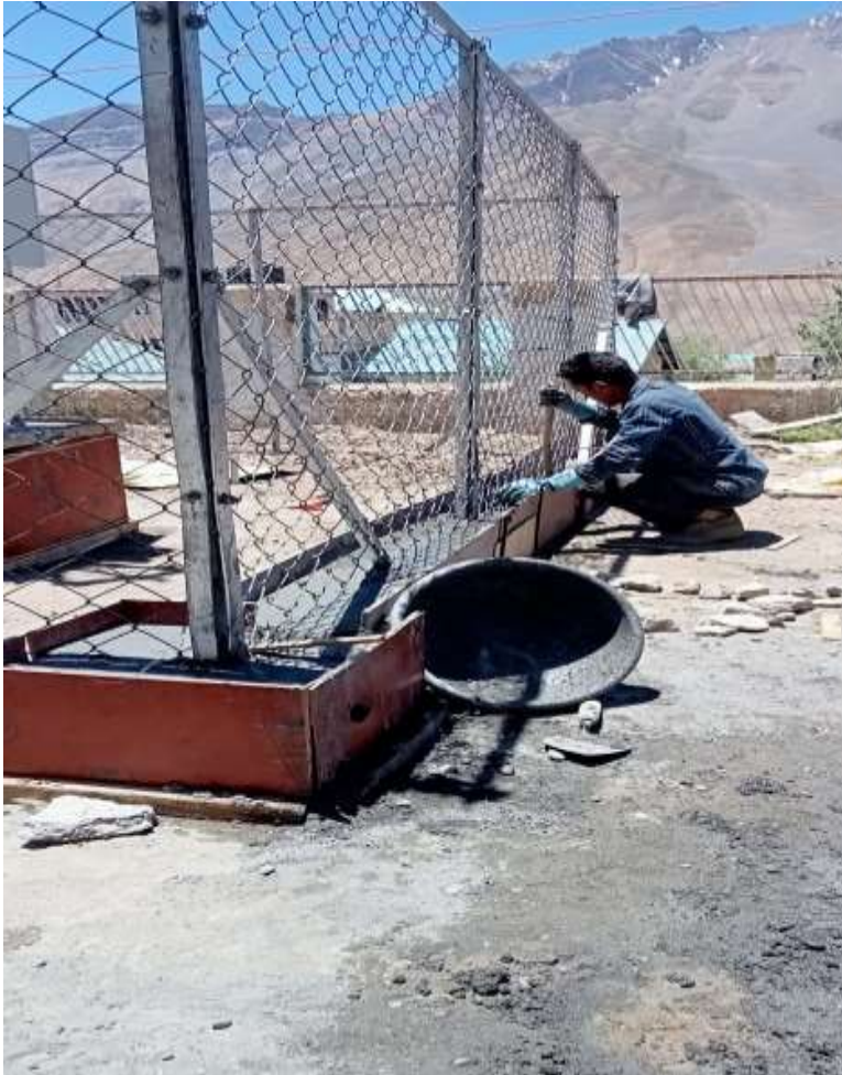
ARG CHAIN LINK FENCING WORK
